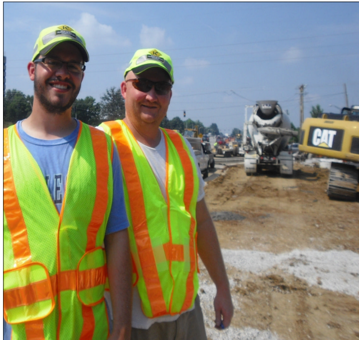
Nathan Wilkinson, Geodatabase Coordinator, with Keith Walker, District 7 Construction, during a concrete pour on the Harrodsburg Road Project.
